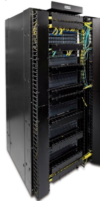
patch location rack
